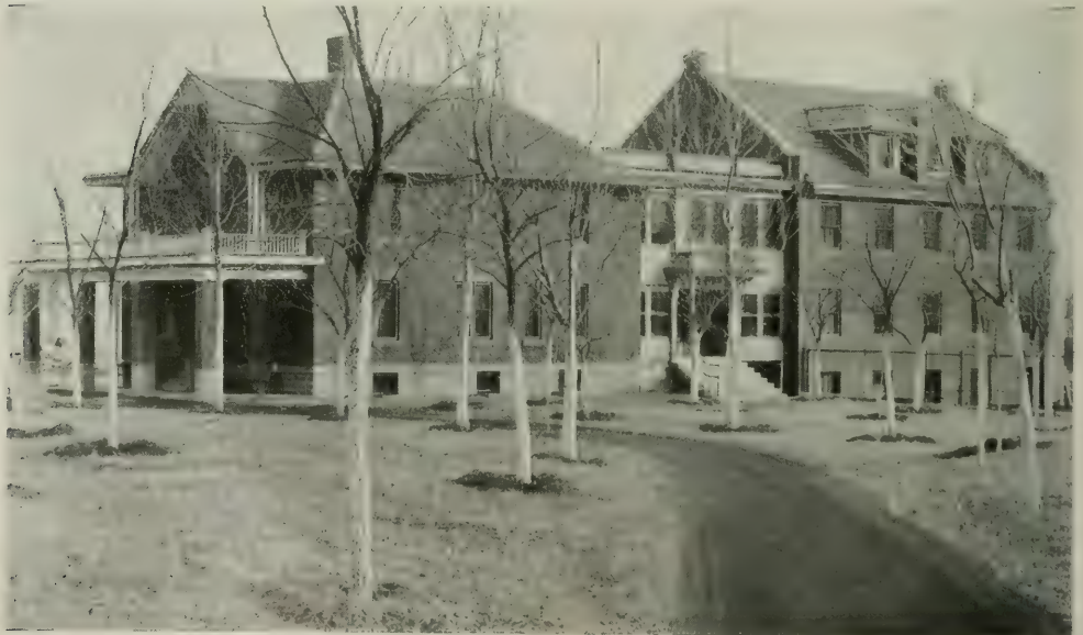
Fig. 3. Green Gables. Rest Cottage.
